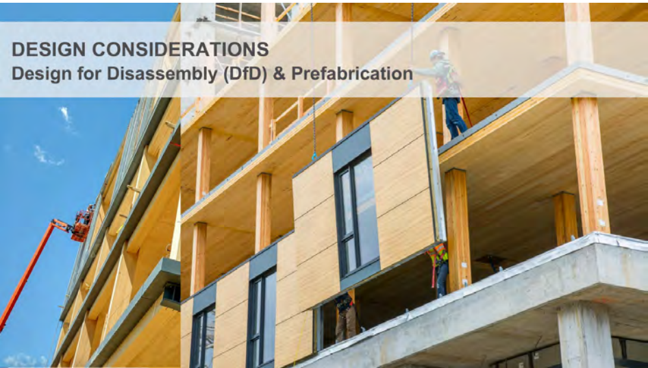
Figure 25. Prefabricated wall panel construction.
