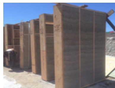
Figure 2. The Marks & Spencer Cheshire Oaks Centre: elevations (left), aerial (center), and a detail of hempcrete construction (right); Cheshire, England; Aukett Swanke Architects.
