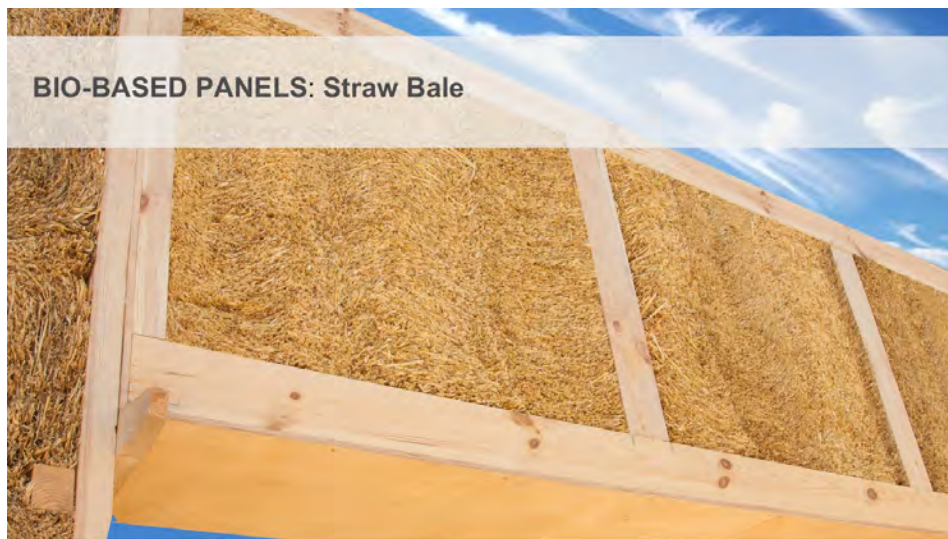
Figure 18. Straw bale prefabricated panel.
